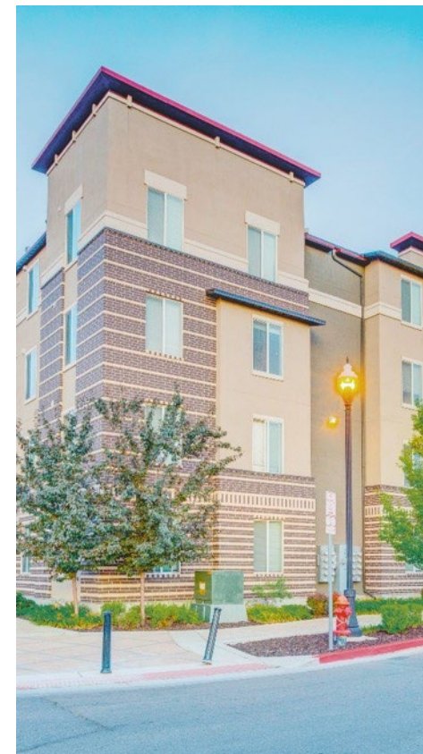
Avida Apartments Multifamily Salt Lake City, UT
