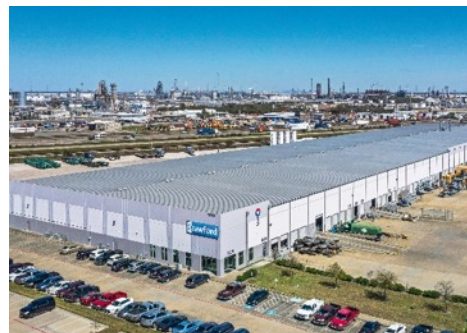
Independence Logistics Park Industrial Houston, TX
